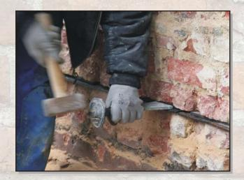
4. Finally fastening the cut joint with static load bearing plastic wedge plates, at a distance of maximum 25 cm over the entire wall cross section (load bearing capacity minimum 500 kg/cm²).
