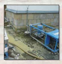
2. Sectional removal of the wall work with PRINZ chainsaw PMS 25, EED 3,5 or PES 1300 for brick walls similarly removal with PRINZ diamond rope saw LP1 for rubble stone or mixed walls. Thus, the length of cut of up to 1,0 m is suited to the constructional and static conditions present.
